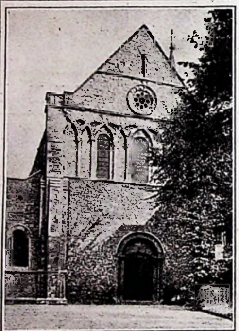
ST. JAMES, BRISTOL, is the old Church of which the Rev. F. W. Potto Hicks speaks in his talk from Cardiff this afternoon. This photograph is of the western facade, and shows the ancient Norman rose window, one of the oldest in England, and the arcade of interlaced arches, three of which are pierced for windows.
